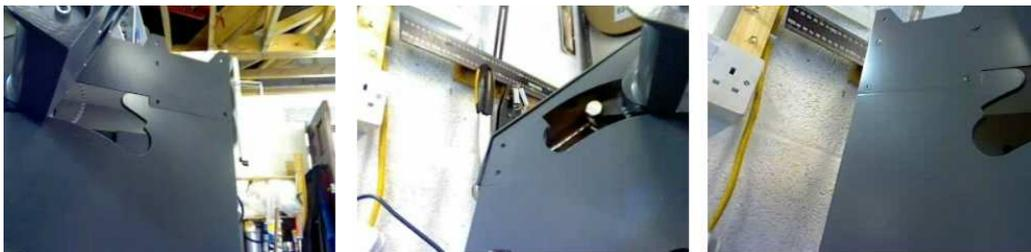
Press the front of the Top Cover down so that it fits neatly against both sidewall panels and the front support piece. Drill a pilot hole through the centre pre-drilled fixing hole and attach using one of the supplied screws. Finish by fixing the two side screws in place.
